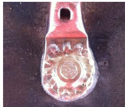
Threaded and Direct types of Pin Braze connections
